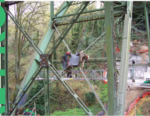
North Queen Anne Drive Bridge
